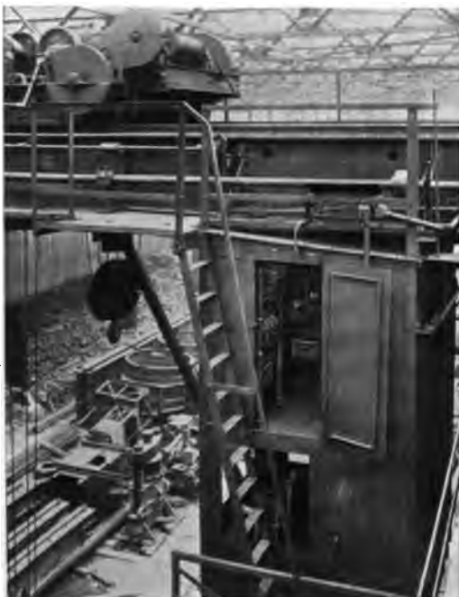
Fig. 3. Crane with Enclosed Double-Deck Cage.
